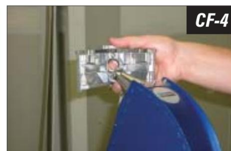
6. Stand directly in front of the internal. It is important to maintain the Tapepro Corner Box nose cone at right angles to the direction of travel and bisect the internal. (CF-5)
